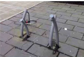
Non-intuitive rack does not provide 2 points of support (Photo: Alta Planning + Design)
